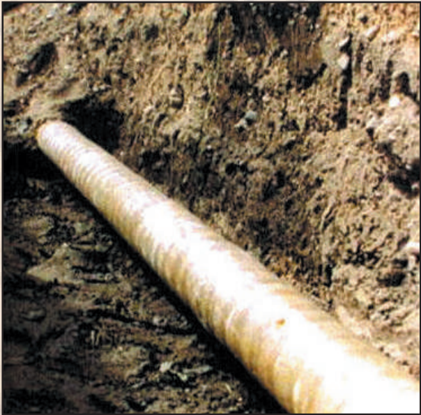
Below ground pipeline can be backfilled immediately
