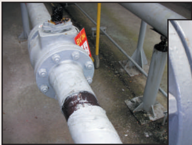
Wax-Tape cut for inspection and repair
