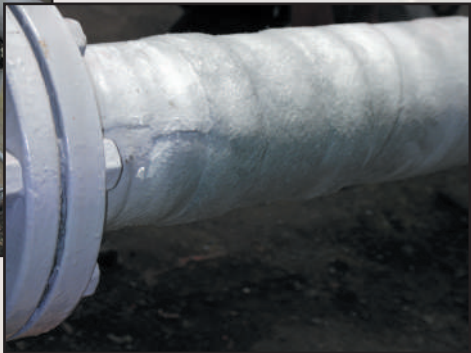
Wax-Tape cut for inspection and repair
