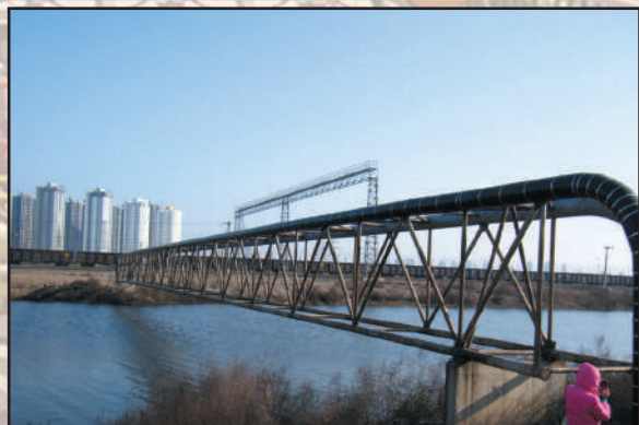
Insulated pipeline across bridge
